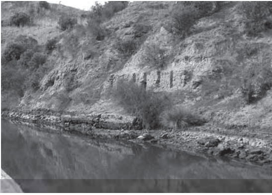
Remains of the Maribyrnong Sand Company's loading chute, Maribyrnong River, Essendon (H7822-0512). Heritage Victoria.
