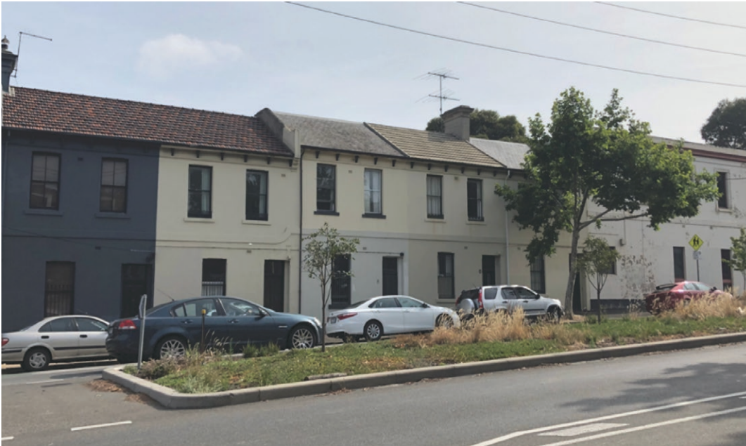
Early terrace row, Arden Street, North Melbourne, Lovell Chen.
